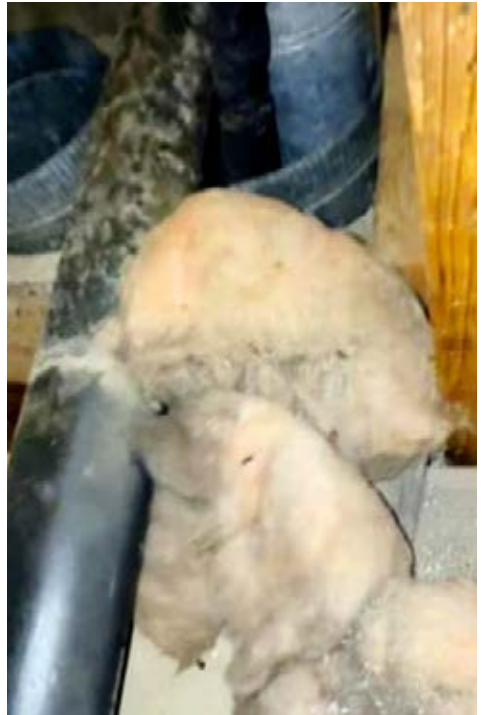
DAMAGE FROM RODENTS THROUGHOUT ENTIRE CONDO
