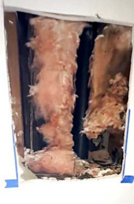
DAMAGE FROM RODENTS THROUGHOUT ENTIRE CONDO
