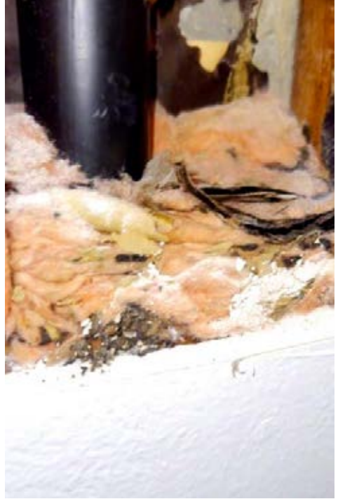
DAMAGE FROM RODENTS THROUGHOUT ENTIRE CONDO
